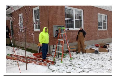
**Repairs and Upgrades** It has been a busy week. Rui from Valley Restoration repaired the water-damaged plaster in the Narthex, then repainted the north wall and insides of the doors. Above: electricians from Comalli are installing the new 400-amp feed at the back corner of the building.
